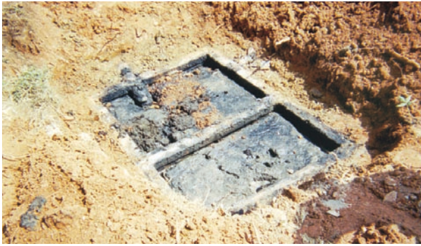
This septic tank was completely filled with solids. Cooperators removed the solids and replaced the tank.
