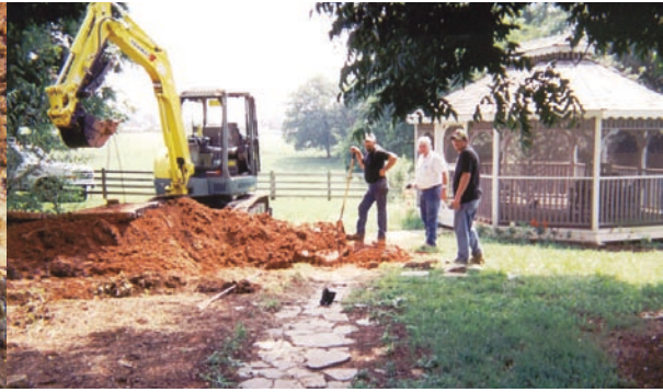
This septic tank was completely filled with solids. Cooperators removed the solids and replaced the tank.
