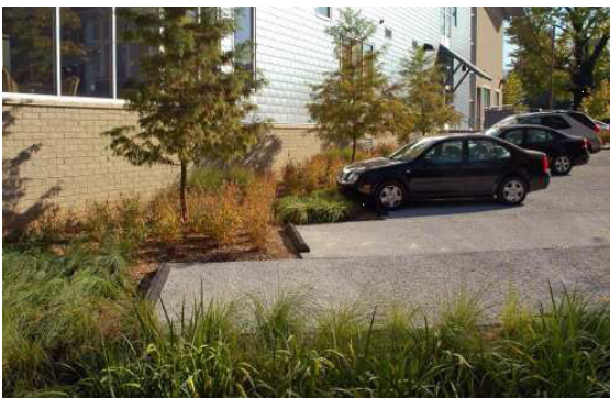
Pervious concrete parking at Tennessee Association of Realtors.
