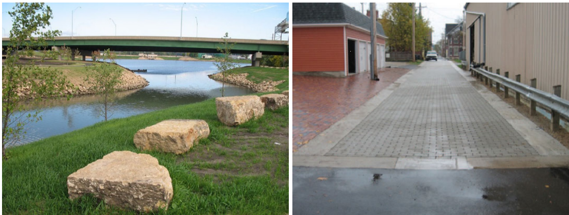
Restoration of Bee Branch Creek (left), and permeable pavement installation (right).
