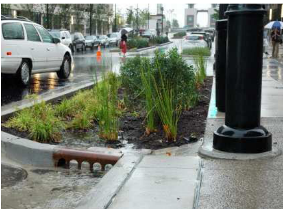
Bioretention area along Deaderick Street.
