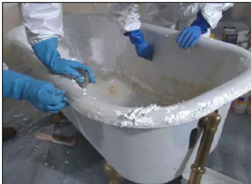
Above: Removing paint from a bathtub (California Dept. of Public Health).
