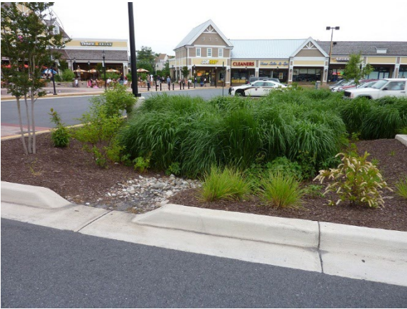
A rain garden collects and treats parking lot runoff in this commercial shopping center in southern Maryland.
