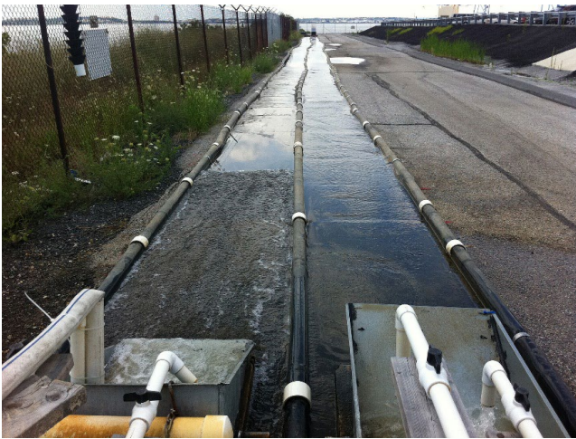
Figure 2. The Algal Turf Scrubbers project is a retrofit solution for treating nutrient-impaired waters. The system relies on native filamentous algae to remove nitrogen and phosphorus from the water as it flows along a raceway. The algae is harvested and used as a cogeneration fuel source at an incinerator.
