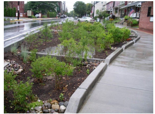
Figure 4. The city of Lancaster included curb extensions and rain gardens in its award-winning ultra-urban BMP project to increase pedestrian safety and treat stormwater runoff. The permeable parking spaces are visible in the background.
