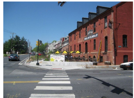
Figure 3. The city of Lancaster, Pennsylvania, implemented the grand prize-winning redesign of the Plum and Walnut Intersection at the Lancaster Brewing Company. The city removed a designated turn lane (left photo) and used the new space for rain gardens, a permeable patio and permeable parking spaces (right).
