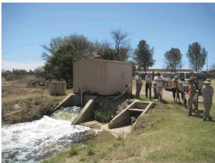
Treated wastewater from the Nogales International Treatment Plant in Arizona flows to the Santa Cruz River.
