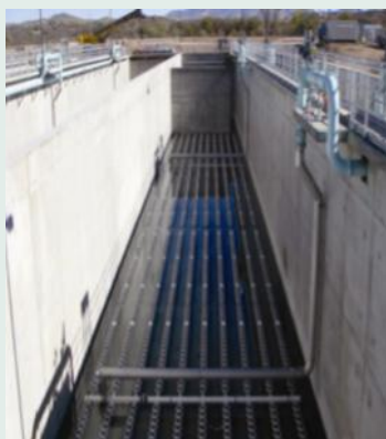
Nogales, Arizona International Wastewater Treatment Plant
