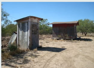
Conditions prior to project implementation
