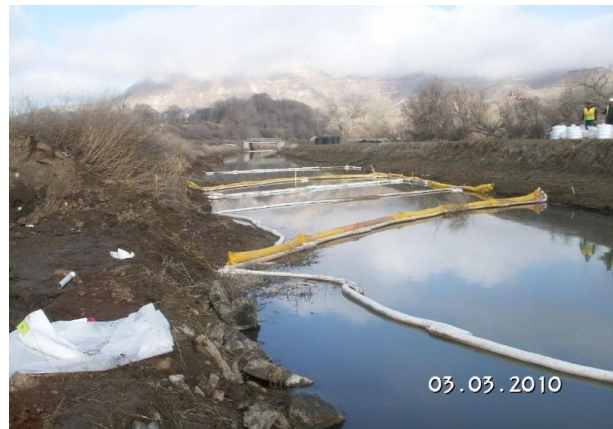
Exhibit 18: Booms deployed to contain and collect diesel spilled by a farm in Oregon in February 2010.
