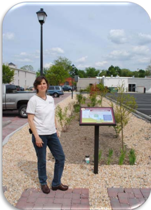
The Retrofit: Ashland’s Town Engineer stands in the parking lot’s new bioretention island. The section at right remains as an asphalt lot.
