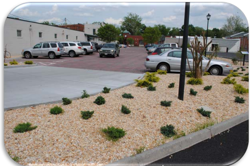
Multipurpose Lot. The multifunctional municipal parking lot demonstrates that stormwater management can be attractive and functional.
