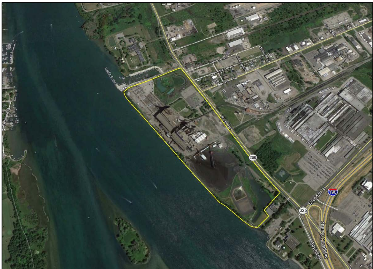
Figure 2-1: Aerial Photograph of Huntley Generating Station
