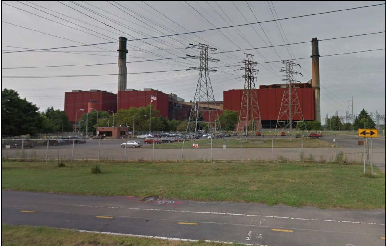
Figure 2-2: Photograph of Huntley Generating Station
