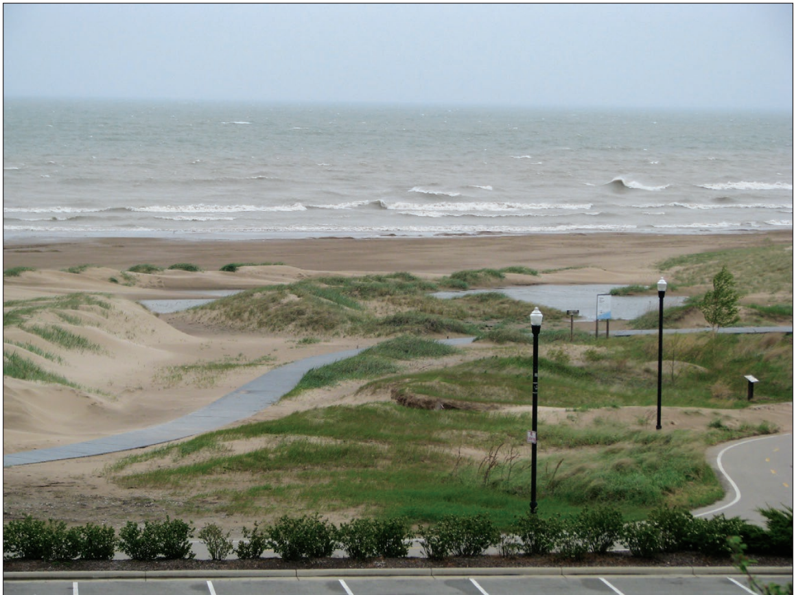
Stormwater retention management practices at North Beach.
