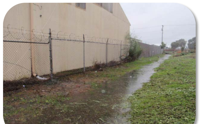
Image depicting the bioswale site after a typical storm event. (Photo courtesy of the Watershed Project)
