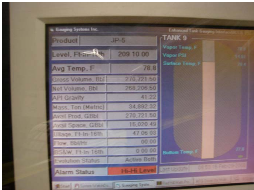
Photo 2 Tank 9 ATG on Feb 29th 2008 at 8:53 am (note level is 209' 10")
