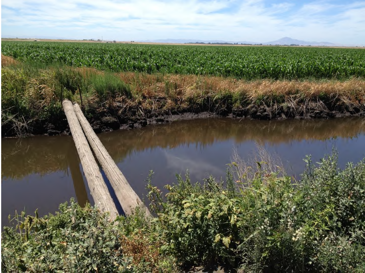
Figure 2-16 Staten Island 1 drainage channel for pasture and alfalfa fields. This is the drainage channel for Staten Island 1 pasture and alfalfa fields. Picture is from sampling event taken place on 6/30/14. Photo shows the drainage channel. The blue arrow indicates the approximate location of the sampling.
