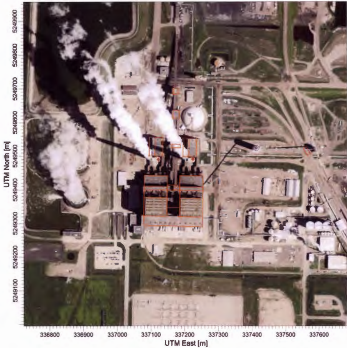
Figure 3-3: Stacks and Buildings Used in the GEP Analysis for Coal Creek Station
