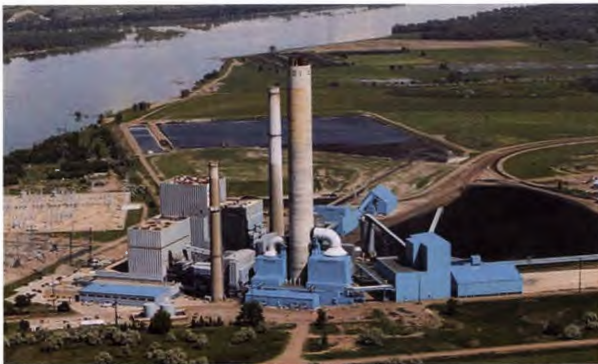
Figure 2-1: Leland Olds Station Photograph
