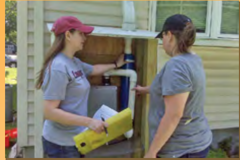
Home vapor mitigation system inspection.
