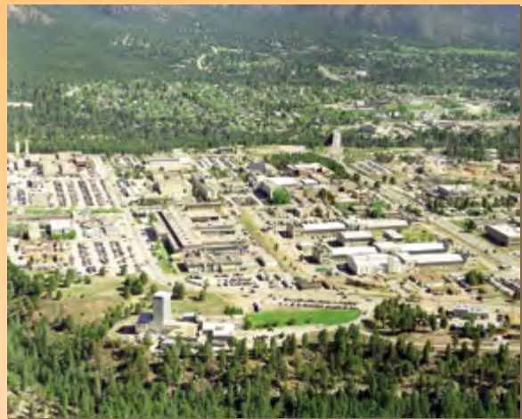
Aerial view of the site. Photo courtesy of Los Alamos National Laboratory.
