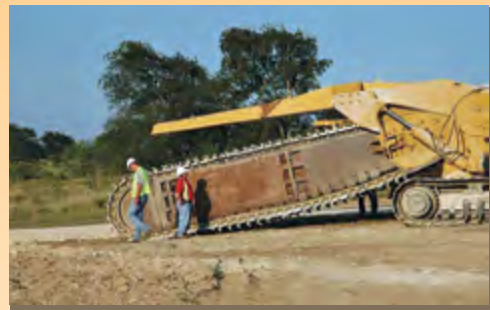
Trenching machine used in biowall construction.
