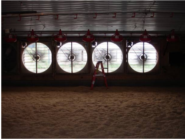
Figure 6.3. Tunnel fans and box air inlets representative of typical southeastern broiler facilities.
