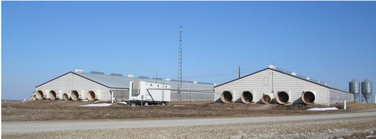
Figure 1. Typical barn monitoring site with instrument shelter between two monitored barns.
