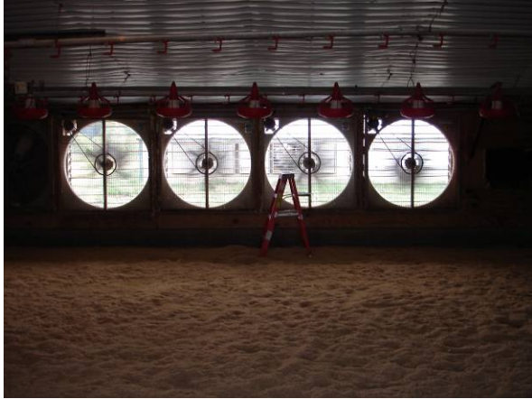
Figure 3. Tunnel ventilation fans and static pressure-controlled box air inlets representative of typical southeastern U.S. broiler facilities.
