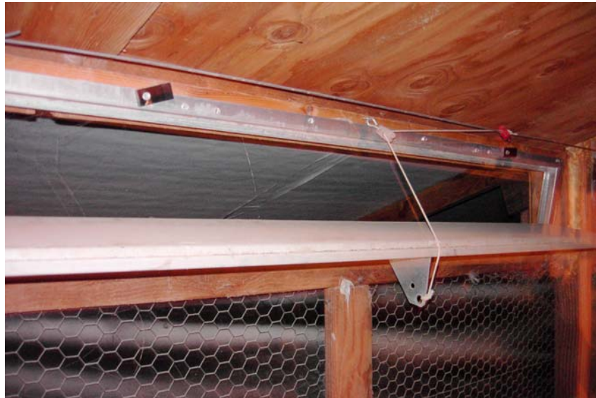
Figure 2. Air inlet in the eave of the barn.
