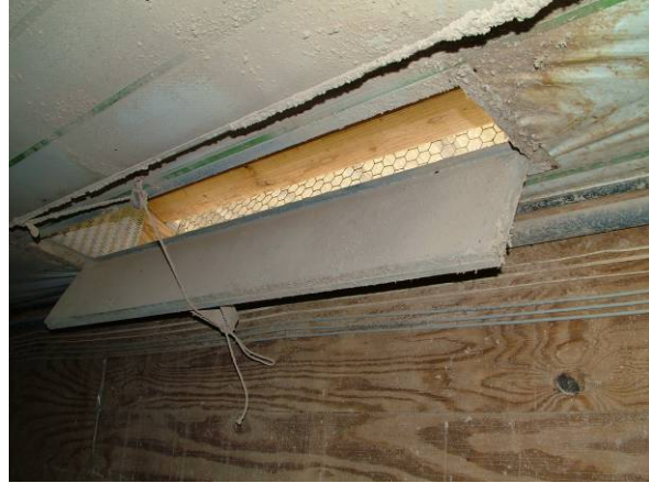
Figure 3. Tunnel ventilation fans and static pressure-controlled box air inlets representative of typical southeastern U.S. broiler facilities.
