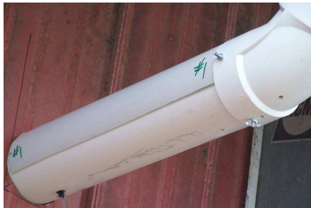
Figure 3. Using a cut piece of thin-wall pipe as a raceway cover.
