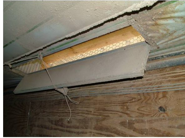
Figure 6.3. Tunnel fans and box air inlets representative of typical southeastern broiler facilities.
