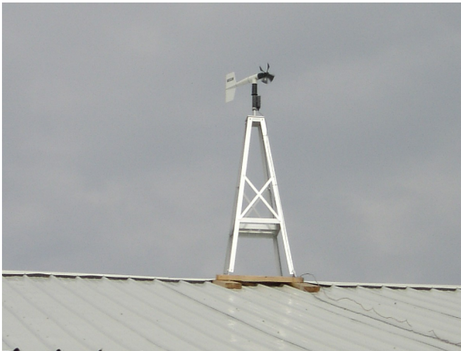
Figure 1. Weather station tower installation on a barn rooftop.
