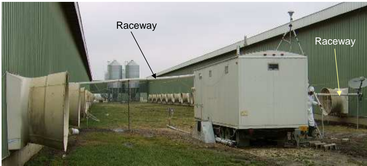
Figure 1. Typical configuration of the OFIS and raceways leading into two barns.
