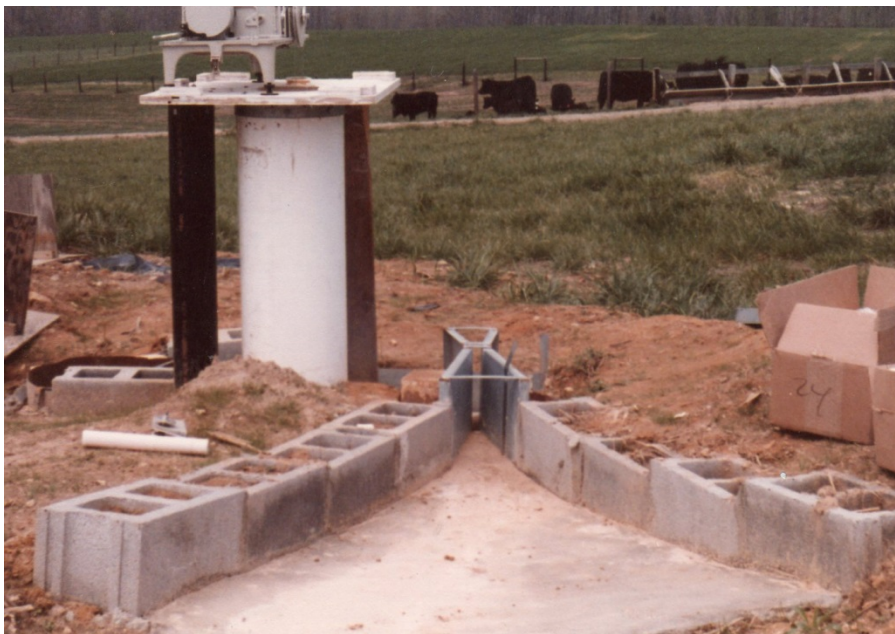
Figure 3-4. Field application of small Parshall flume
