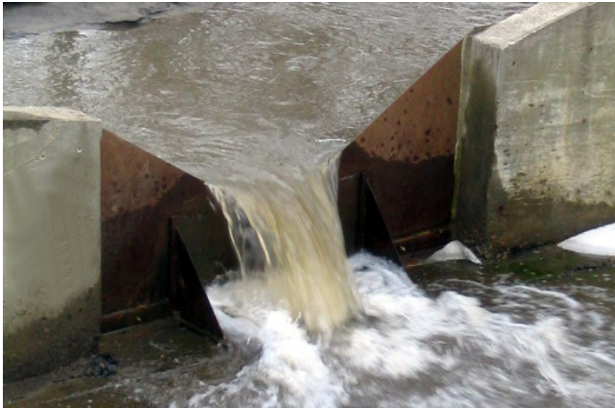
Figure 3-3. 120° V-notch weir, Englesby Brook, Burlington, VT
