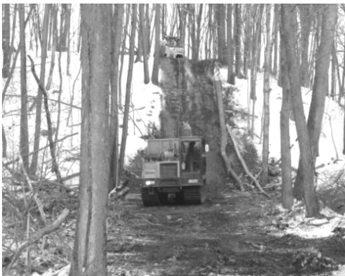
Enbridge cleanup contractors built roads over frozen ground in environmentally sensitive areas near Talmadge Creek and the Kalamazoo River.
