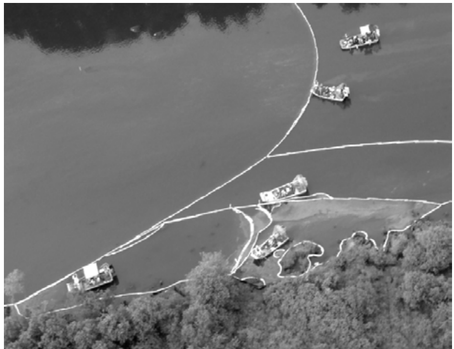
Sediment agitation frees submerged oil so it can be collected, removed and sent off-site for disposal.
