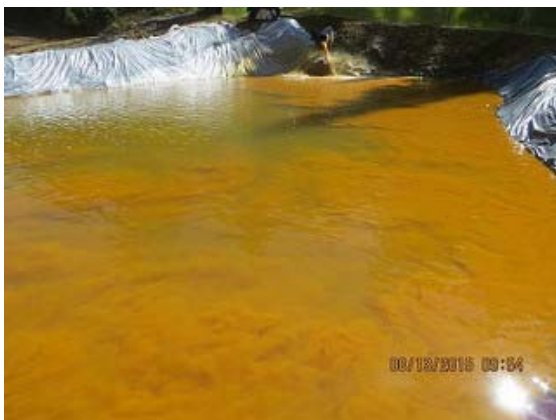
Yellow boy formation with acid neutralization in a treatment pond
