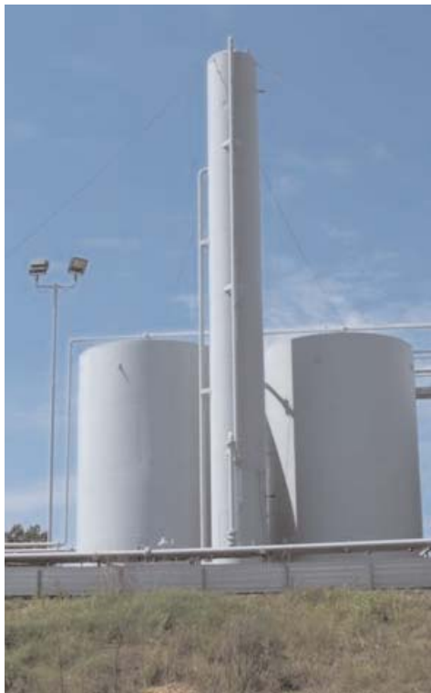
Vapor Recovery Tower. Photo Courtesy of Anadarko.
