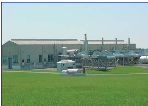
Midwestern Gas Transmission Company's Portland Compressor Station located near Portland, Tennessee.
