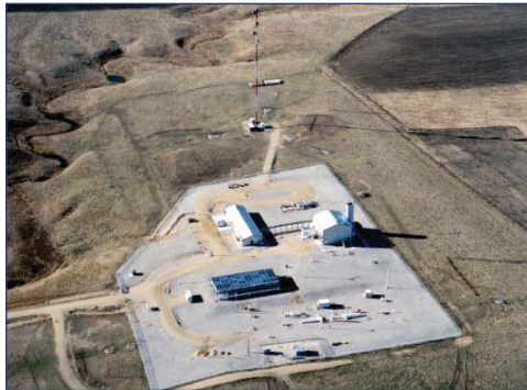
Northern Border Pipeline Company Compressor Station No. 11 located near Brandt, South Dakota.
