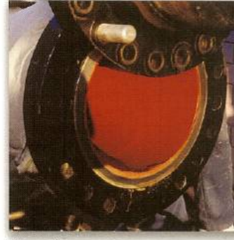
Pipe after coating.
