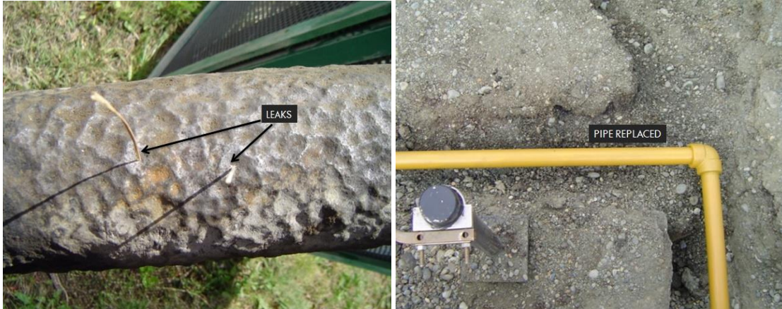
Figure 5. Photos of the Underground Line Before and After Repairs.
