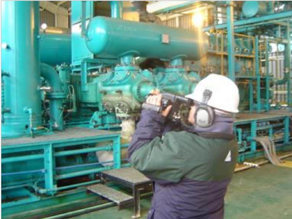
Figure 8. Technician Performing Inspection Work.
