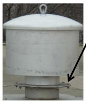
For elevated tanks, having fewer than 8 inches from the bottom of the #24 mesh to a horizontal surface will trigger a significant deficiency
