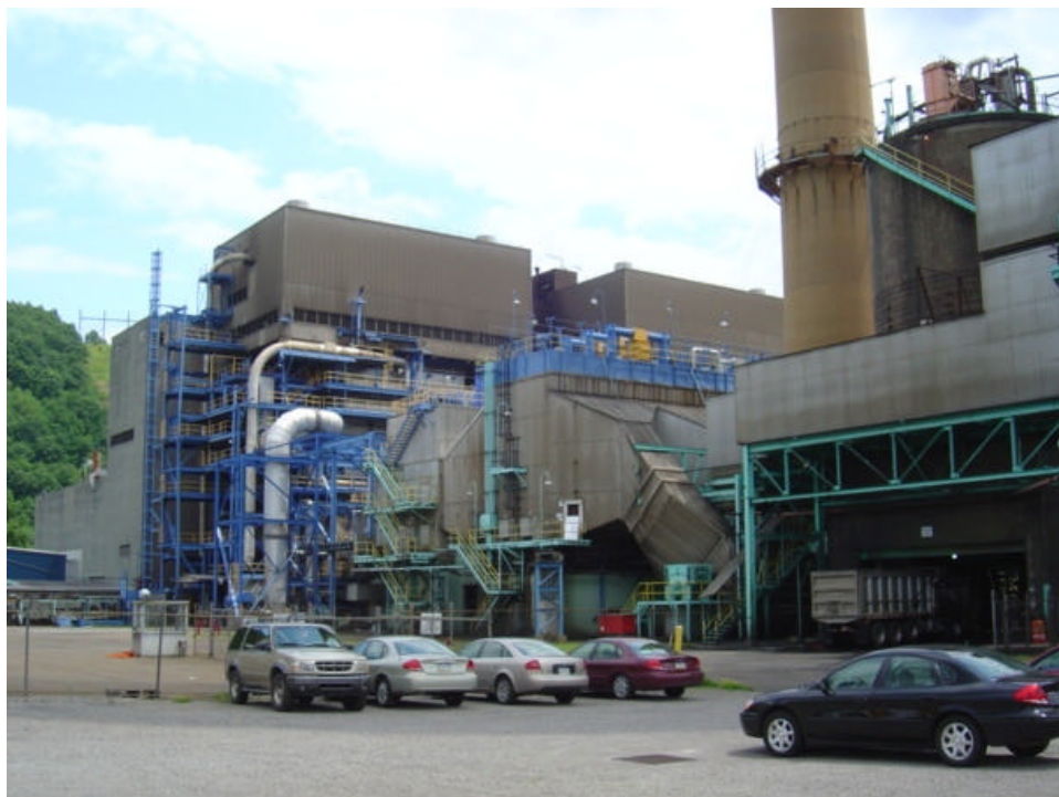
Figure 3-4: ESPs at Armstrong Unit 3
