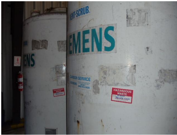
Photo #21: Portable tanks holding hazardous excess recycle water in the IS container storage area.
