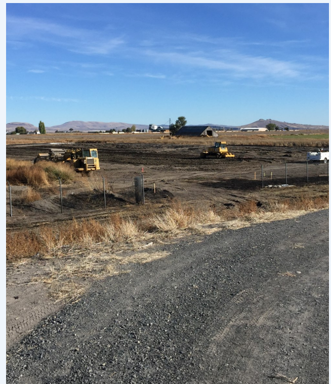
Breaking ground for a new recycled water system
