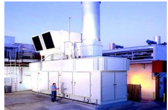
Mark McDannel, LA County San
