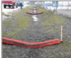
Installation of filter socks in a road ditch by Earth Corps for Indiana Department of Transportation. The filter socks will be staked through the center. Source: Filtrexx International, LLC.
