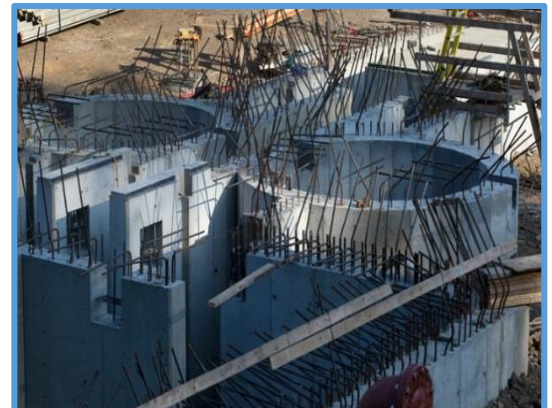
Martinsburg plant during construction. Photo Courtesy: HRI Inc.
