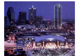
Redevelopment—either through clean up or engineering controls, property is ready for productive use
