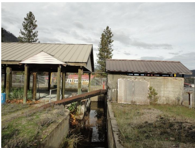
Influent from Sand Settling Basin pumped to two locations (on a Y diversion)
