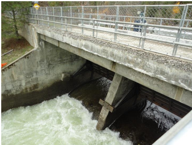
Structure 2 –upstream of the Hatchery – gate stays open to leave water in Historical Channel of Icicle Creek – not running water over the Hatchery Channel
