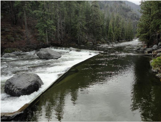
LNFH Intake on Icicle Creek – Overflow, sediment settling, canal into Intake House below
