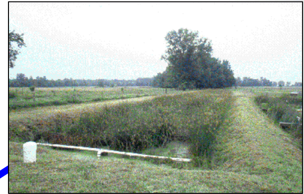
Constructed Wetland Effectiveness Agricultural Watershed, OH
