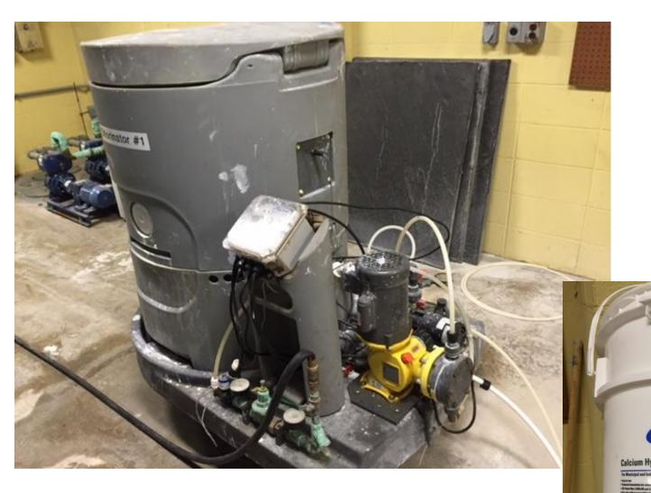
Calcium hypochlorite feed system used at Westside and Cedar Street Reservoirs prior to July 2016. Contributed to the wide swings in chlorine levels.
