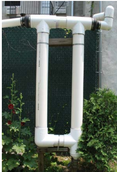
Exhibit 14-11. Roof Washer (Credit: NCSU BAE)
