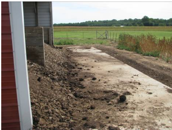
Photo 17-2. This storage structure might have inadequate capacity for the amount of litter being stored. The area around the storage shed drains to a water of the U.S. and does not have any runoff controls. (Source: EPA Region 3)
