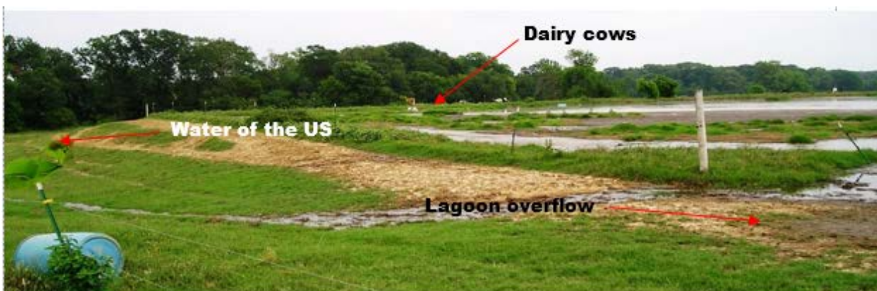
Photo 17-1. This lagoon at a dairy CAFO is upslope from a water of the United States and overflowing. In addition, cows stand on the embankments of the far side of the lagoon, which may degrade the embankments over time, and vegetation is growing in the lagoon, which indicates poor maintenance. (Source: EPA Region 6.)
