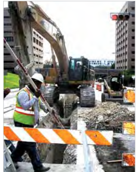
Construction of city-supplied reclaimed water distribution lines
