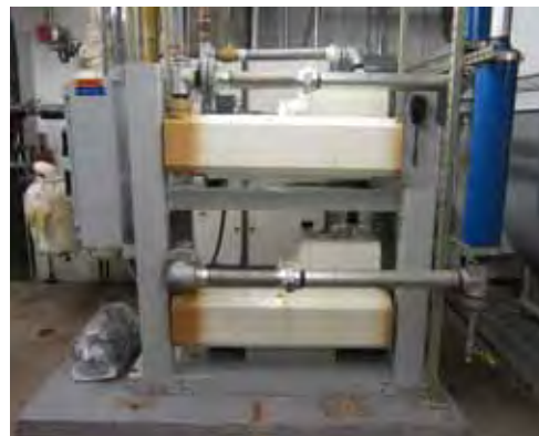
Anesthesia evacuation pumps
