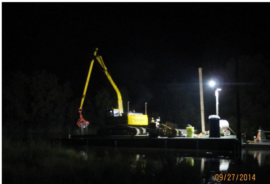
Photo 2. Dredging at night along the South Channel
