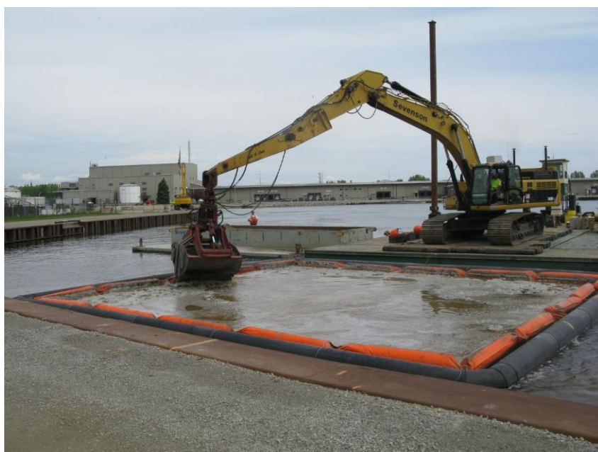
Photo 24. Moon Pool used during cover placement
