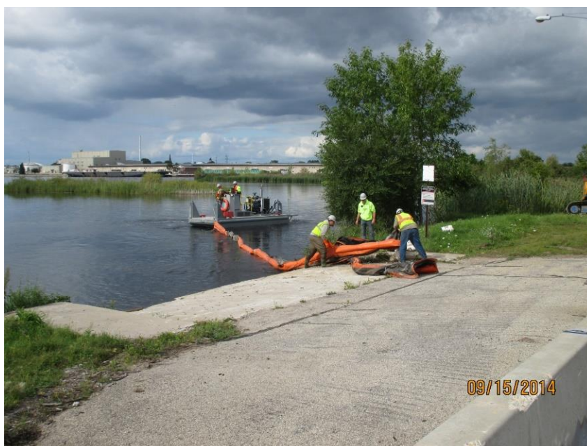
Photo 22. Deploying turbidity curtain for cover placement
