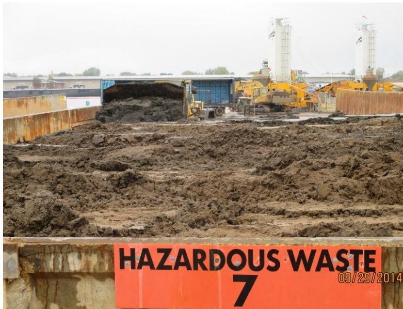
Photo 15. Processing sediment to bin
