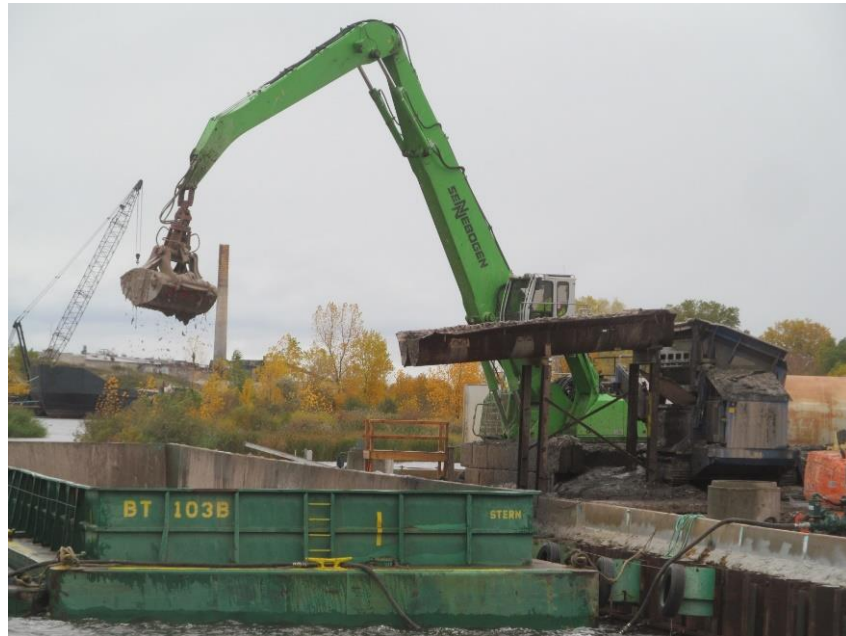
Photo 9. Off-loading Sediment
