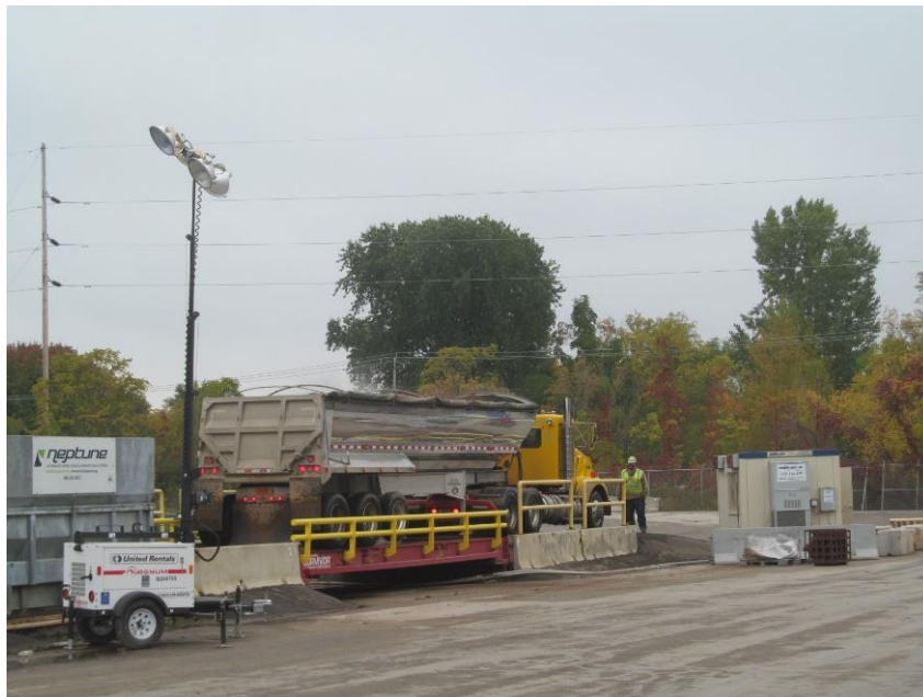
Photo 21. Weighing processed material for disposal
