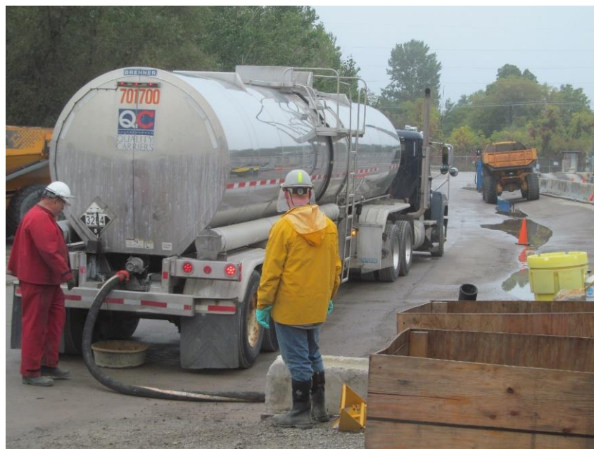
Photo 14. Offloading Liquid Ferric
