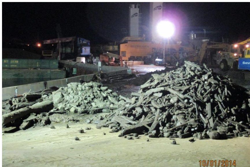
Photo 11. Separating into debris pile
