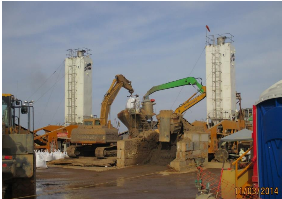
Photo 13. Loading Dry Ferric
