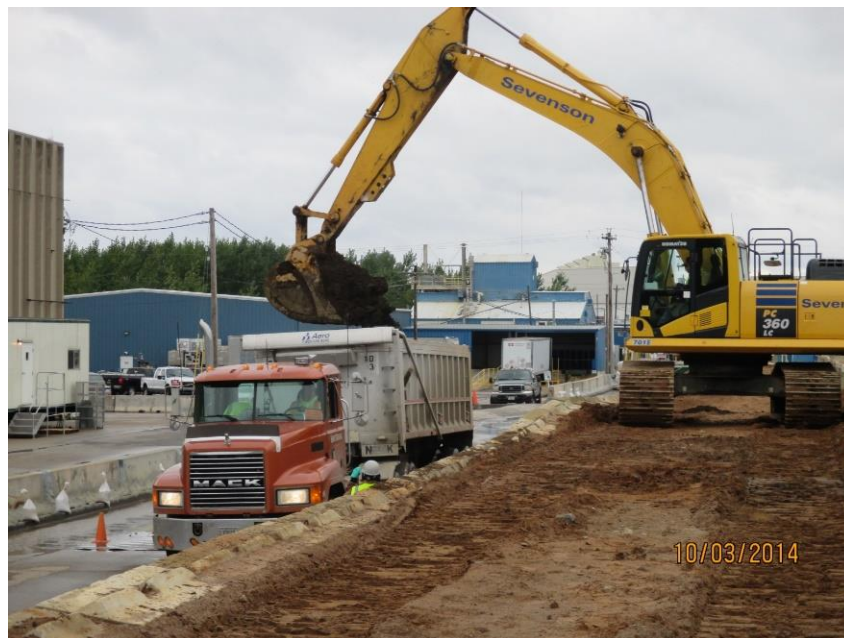
Photo 19. Loading processed sediment for disposal
