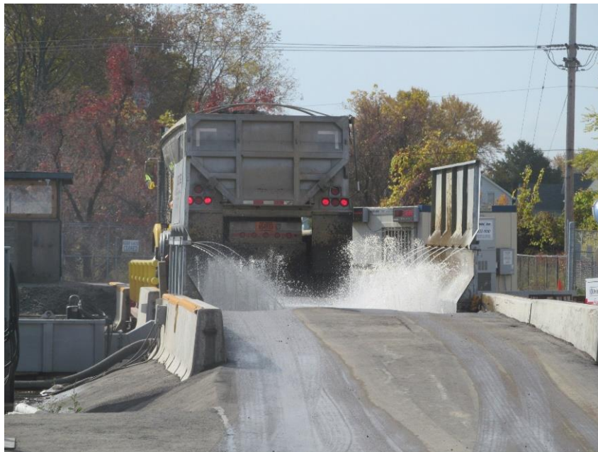
Photo 28. Truck decontamination during the loading out process
