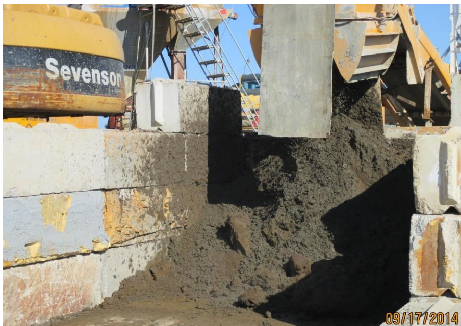
Photo 16. First load of sediment processed
