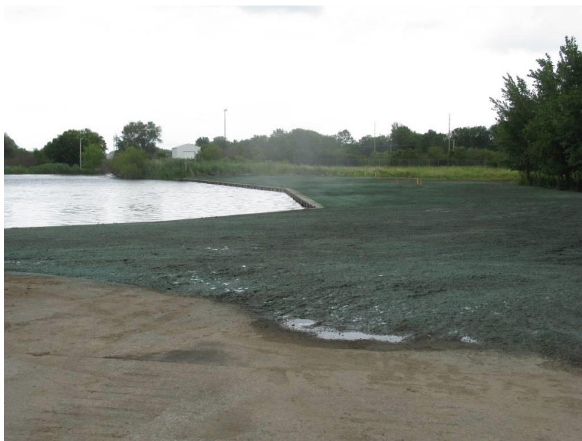
Photo 31. Site Restoration: Wetlands Hydroseeding
