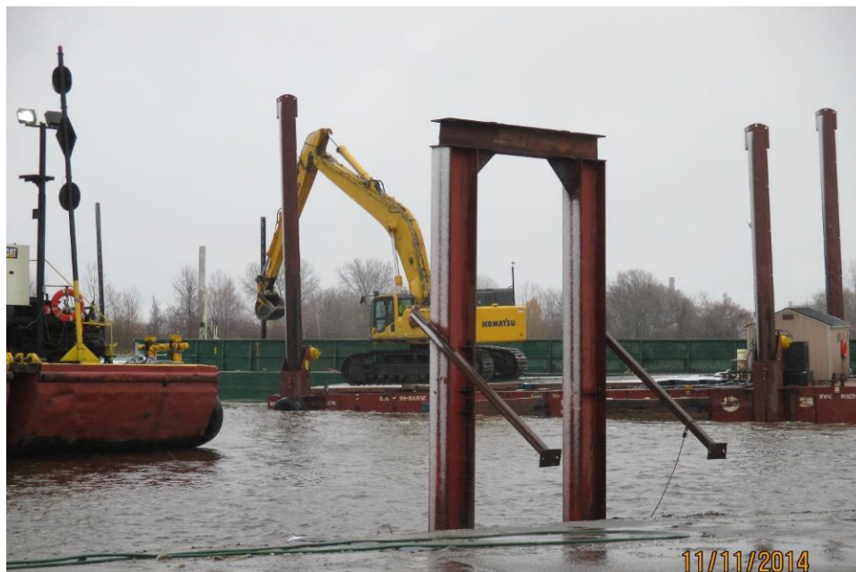
Photo 5. Re-dredging in L8
