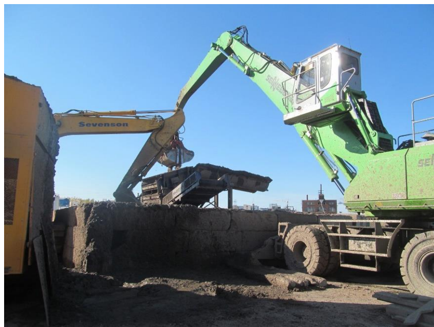
Photo 10. Off-loading and screening of sediment
