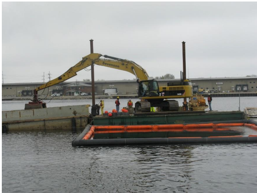
Photo 23. Moon Pool used during cover placement
