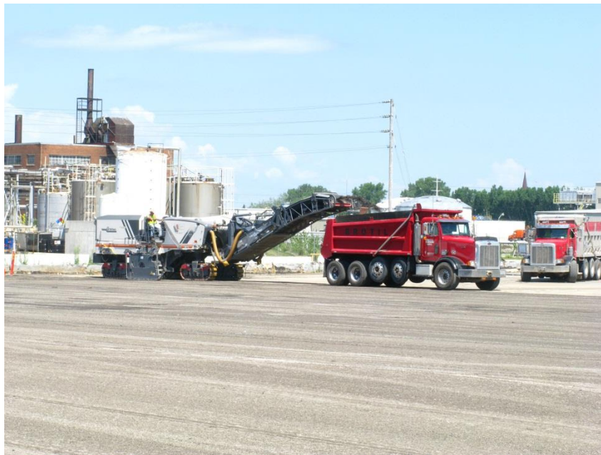
Photo 32. Milling Process Pad
