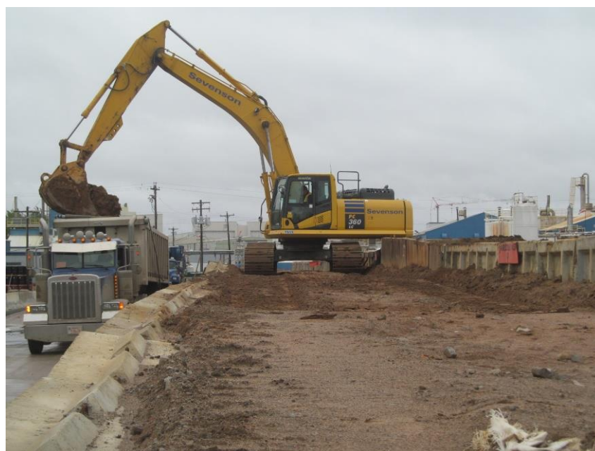
Photo 20. Loading processed sediment for disposal
