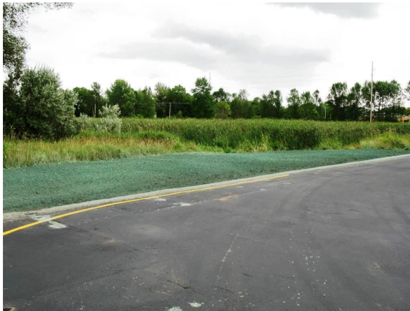
Photo 30. Site Restoration: Hydroseeding at 6th Street
