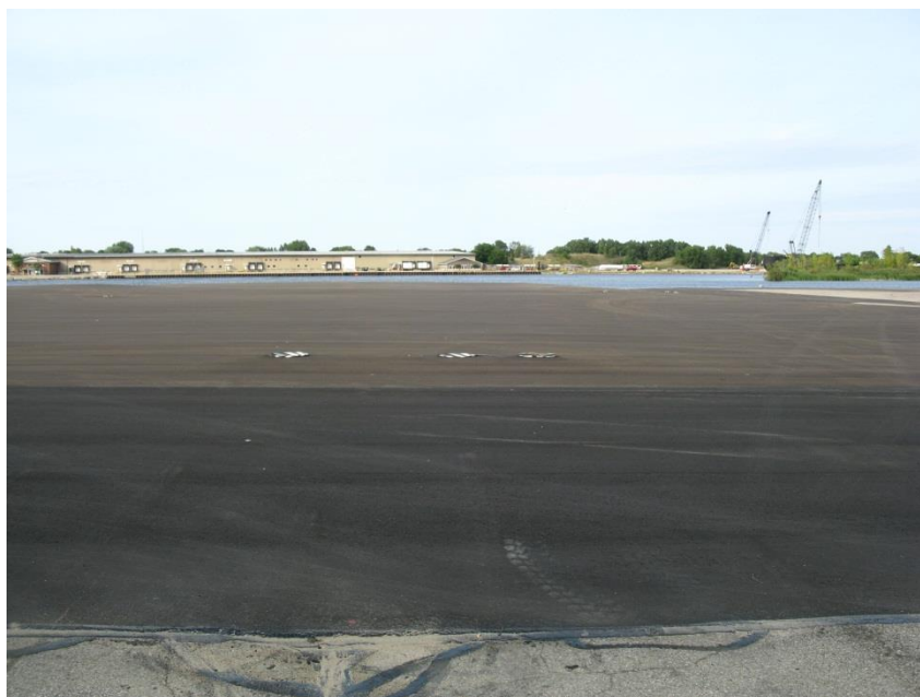
Photo 33. Asphalt Paving Complete
