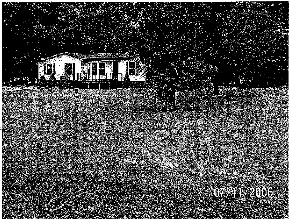
No. 12 Looking northeast at home located on Lot 1209 on Allman St. Location B.
