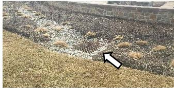
Photo 14-4. If the outlet is set too low, then stormwater will not pond and very little water will infiltrate, as it is designed to do. (Credit: John Kosco, Tetra Tech)
