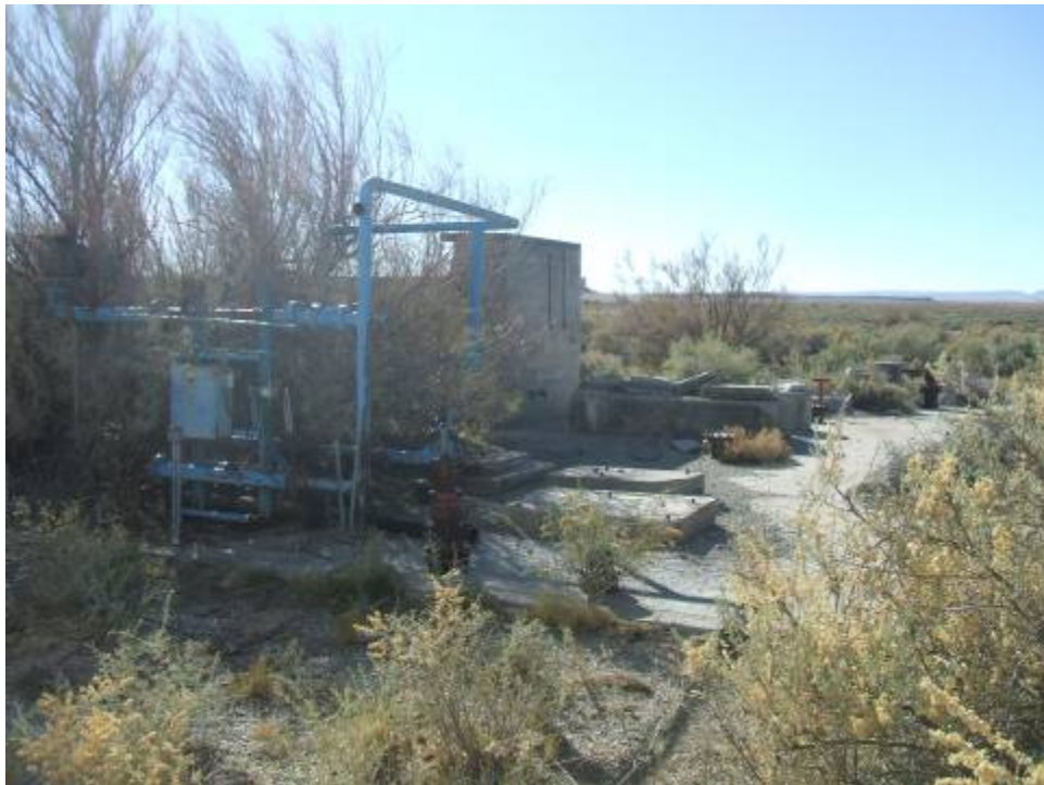
Photo 10. Nose Rock No 1 mine site water pump and well, near northern tank, towards the south
