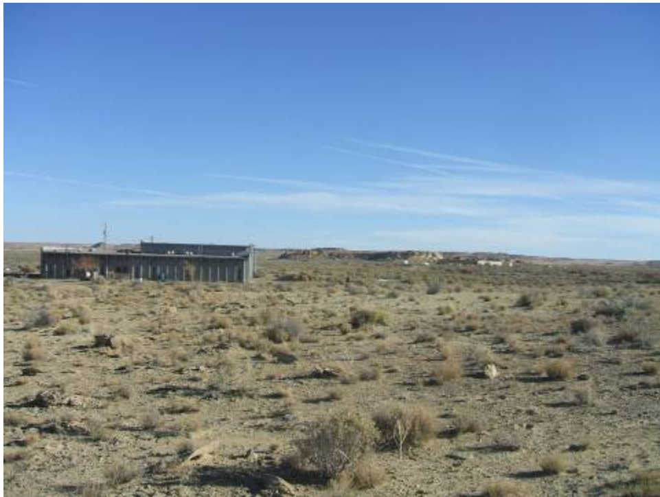
Photo 2. Nose Rock No 1 mine site southwest area building, towards the northeast
