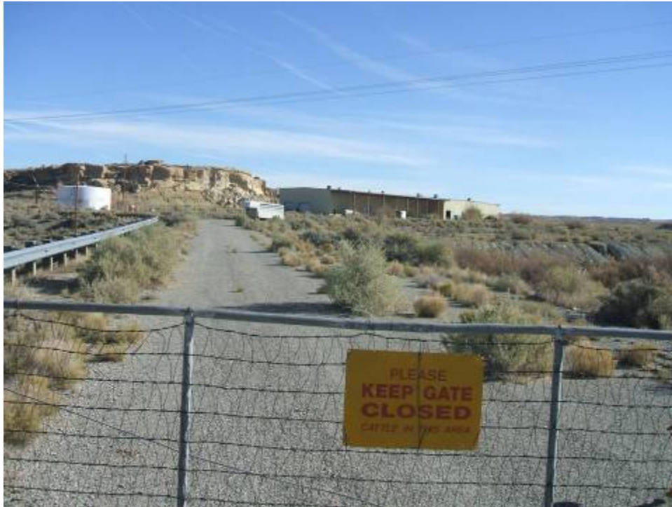
Photo 5. Nose Rock No 1 mine site warehouse building vicinity in northern area, towards the north
