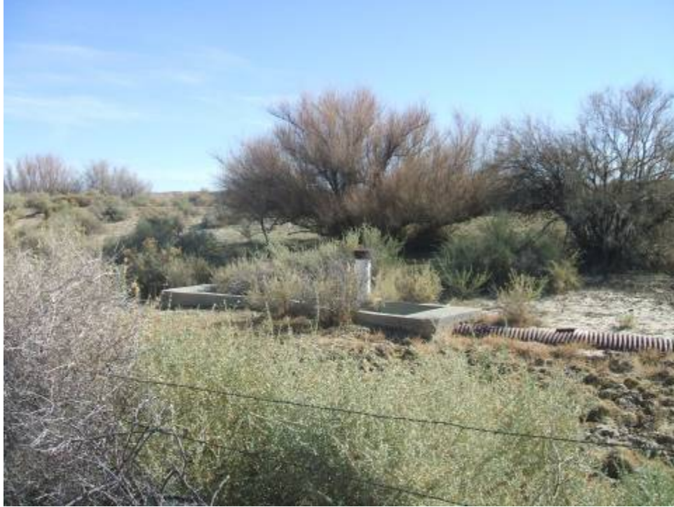
Photo 13. Nose Rock No 1 mine site well and concrete containment in central area, towards the east
