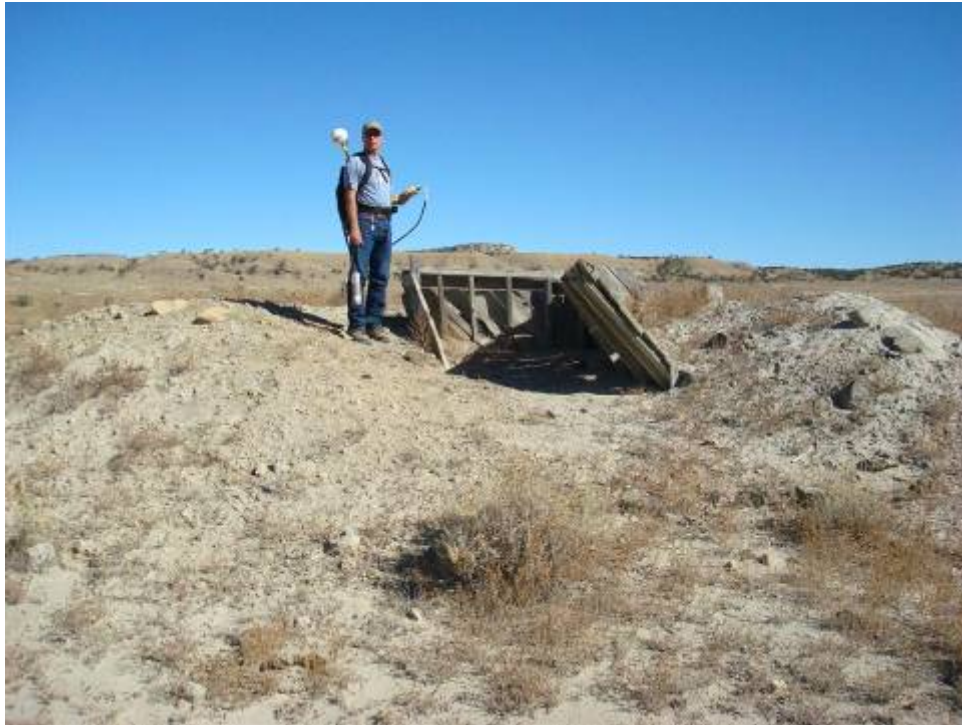
Photo 3. Section 33 Mine site, wooden hopper and pulverized waste rock pile located at southeast corner of mine
