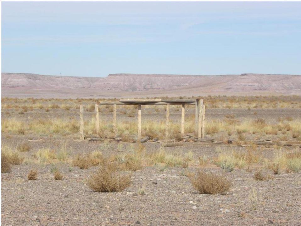
Photo 4. Ryan No. 1 mine site, wood pilings
