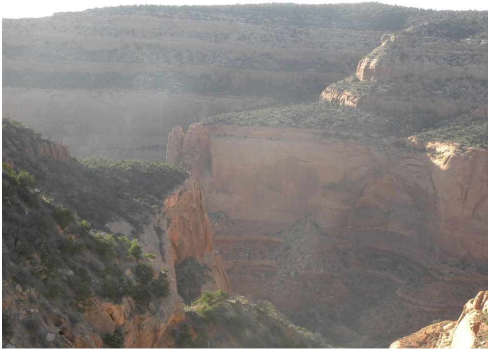
Photo 3. Site #197 – Cliff area and waste debris
