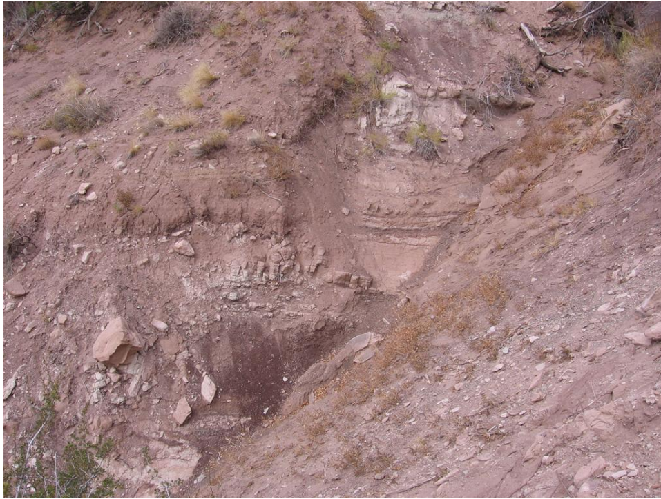
Photo 1. Walking pathway towards mine site washed out
