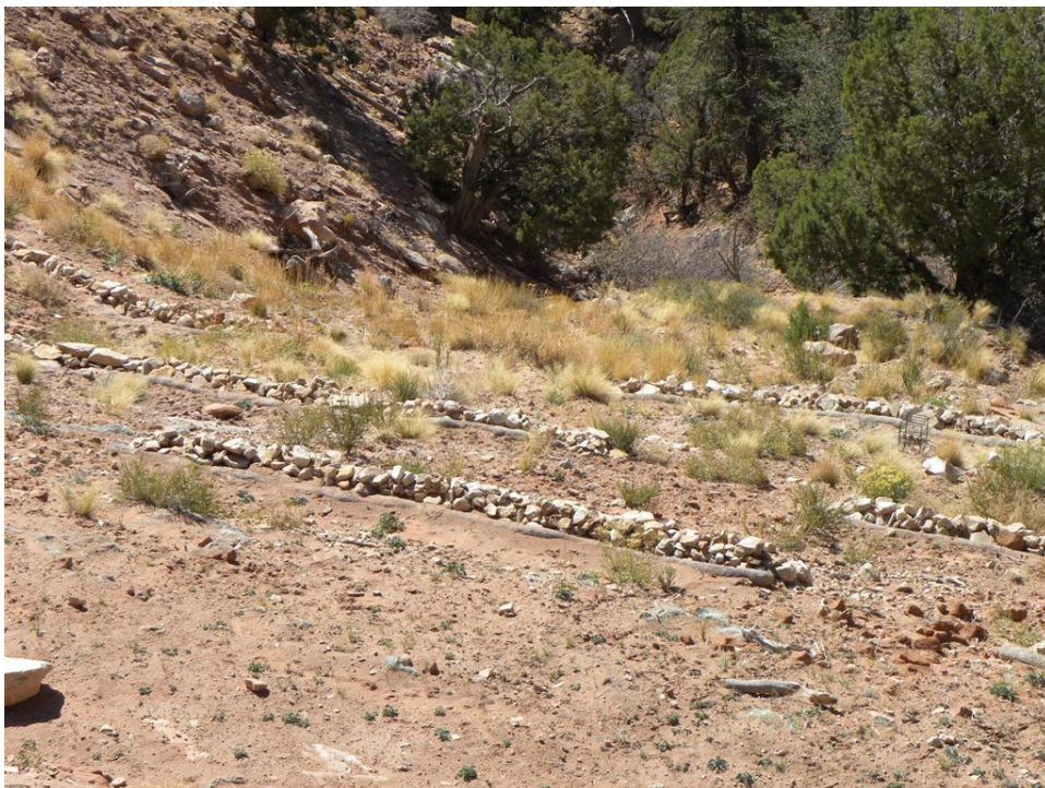
Photo 2. Rip-rap barriers to curb erosion
