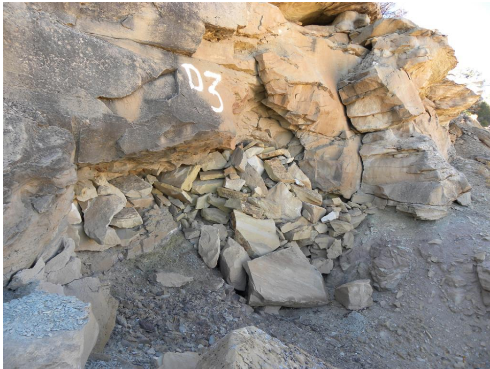
Photo 2. Sealed adit and waste debris
