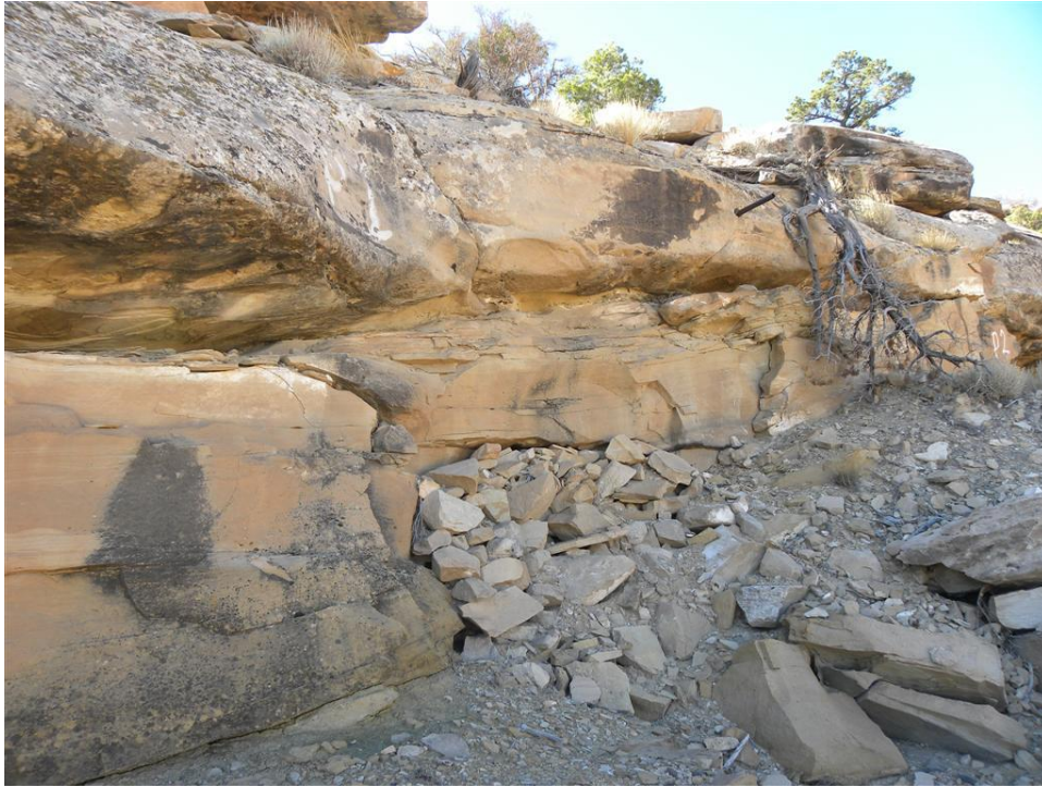
Photo 7. Sealed adit and waste debris
