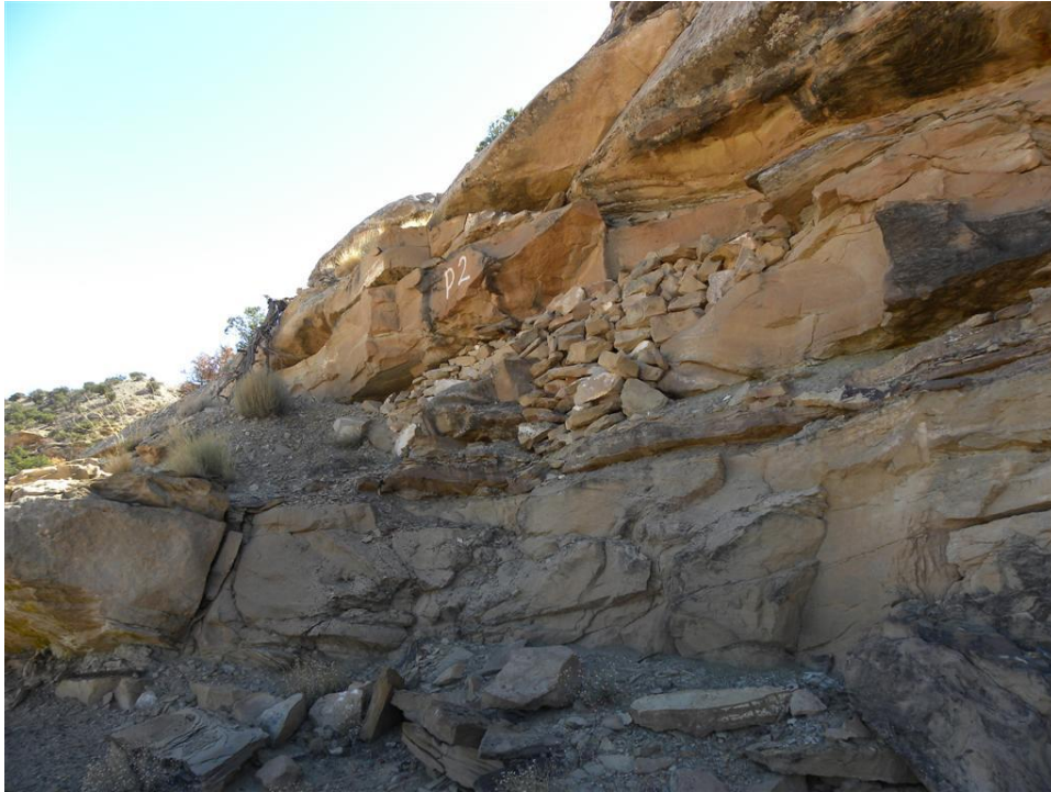
Photo 5. Sealed adit and waste debris
