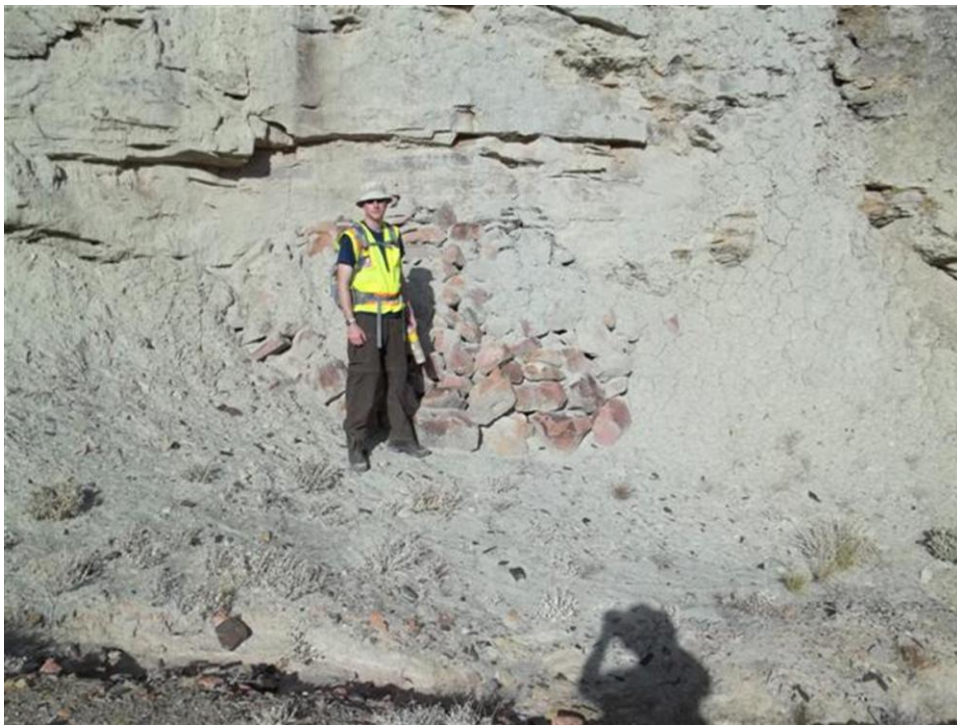
Photo 2: Mine Site #290; Sealed adit
