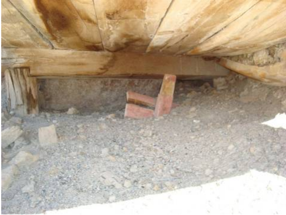
Photo 11. Alta Mine site, adit
