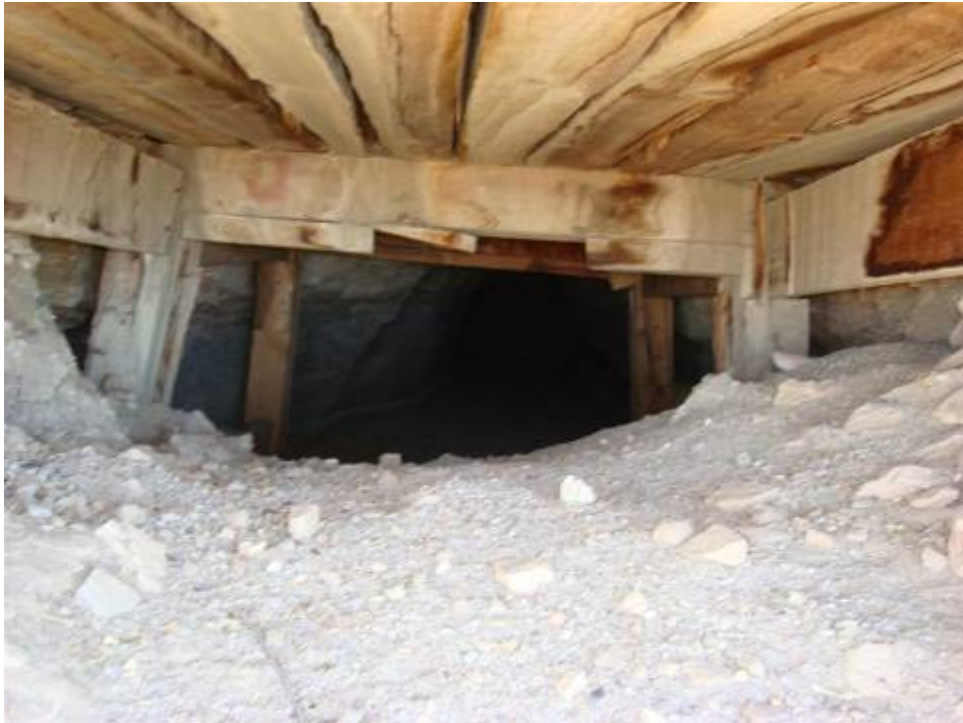
Photo 10. Alta Mine site, adit
