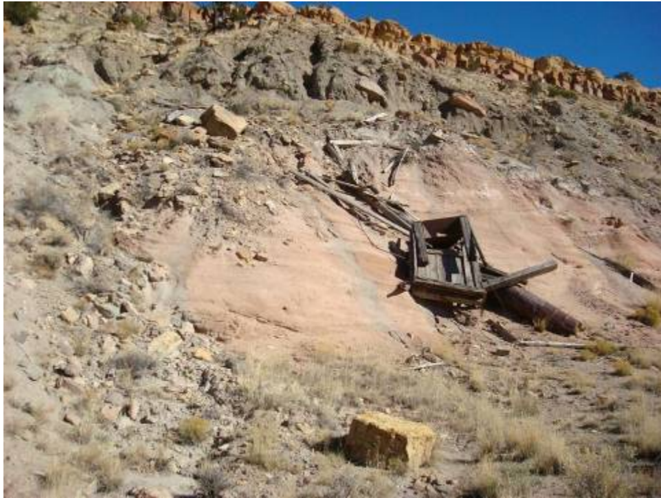
Photo 13. Alta Mine site, collapsed wood structure
